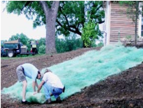
Unroll erosion control blankets from top of slope to bottom and overlap edges to attain complete coverage. Pin down blankets securely.
